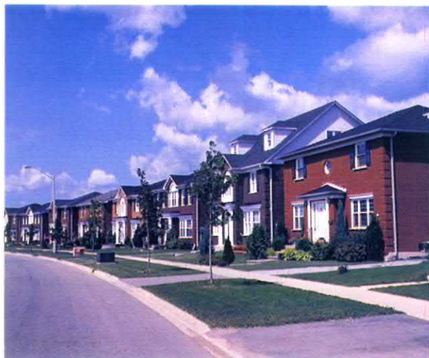
Streets are considered to be part of the public open space network.
