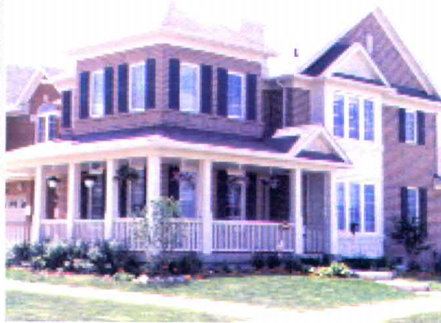
Side elevations equal to the front elevation treatment will be provided on those elevations visible from the street.
