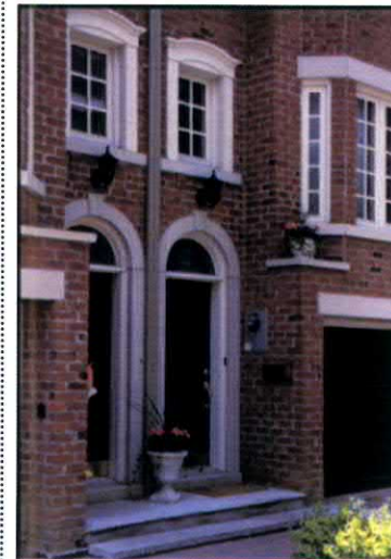
Meters located to reduce exposure.
