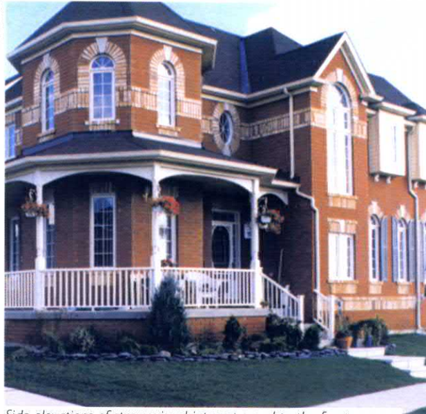
Side elevations of strong visual interest equal to the front elevation will be provided.
