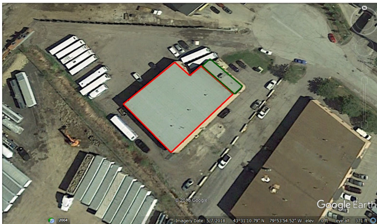
Figure 23 | Milton Transit Facility Building, garage is circled in red and office is circled in green
